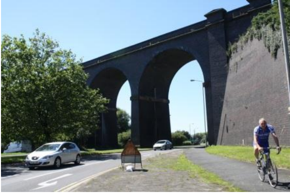
Coming under Kidderminster Viaduct
